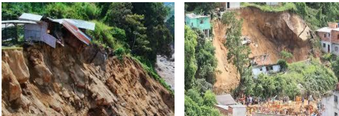
Figure 2. Landslide signs in areas prone to landslides
